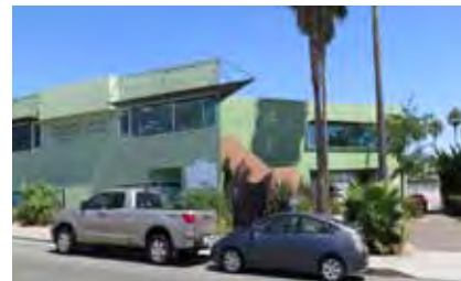
Cardiff's architecture is more eclectic and colorful, and buildings are modestly scaled.
