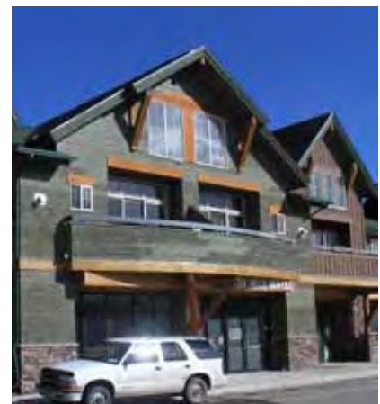
Rustic materials and finishes are part of the design traditions in Olivenhain.
