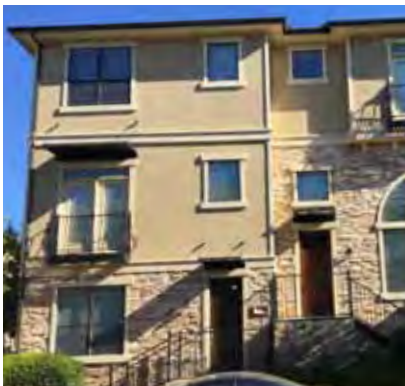
The materials featured in this photo are acceptable in the Old and New Encinitas context.
