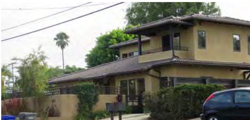
Terrace development on steep slopes, following the natural contours of the site.
